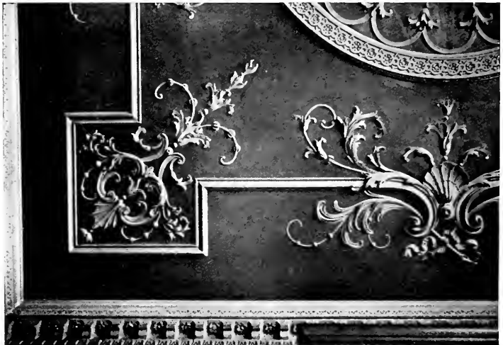
240. Ceiling, 44 Great Ormond Street.
